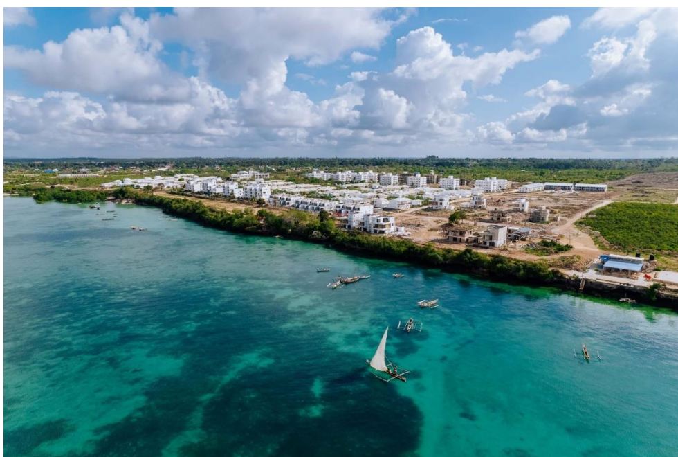
The construction of Fumba Town is on its way
